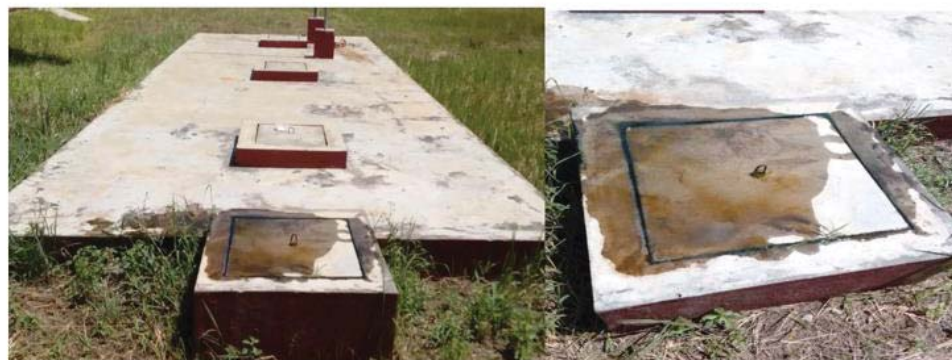
Figure 1: Image of a septic tank overflowing with sewage at FCT-UL, Dondo Campus, March 2024. Source: Author 2024 [10].
